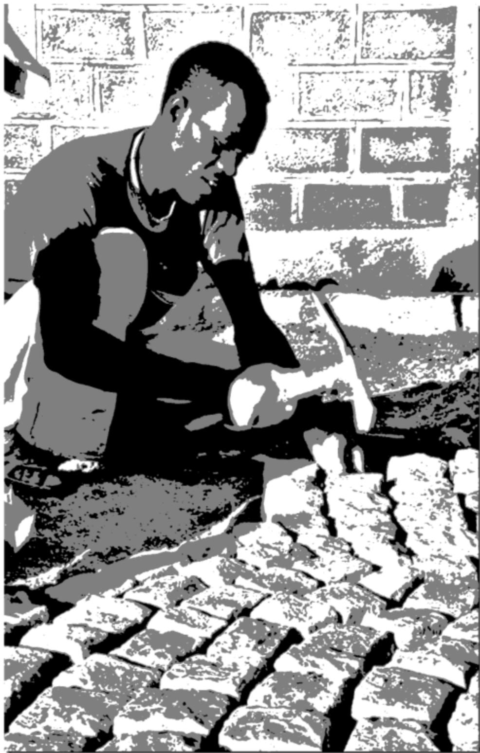
Once the stones are set, the fill between cobblestones is put in place. First the stones are secured using smaller stones as stabilizers (if you have put down pavers, we use little plastic plus signs between machined tiles):
