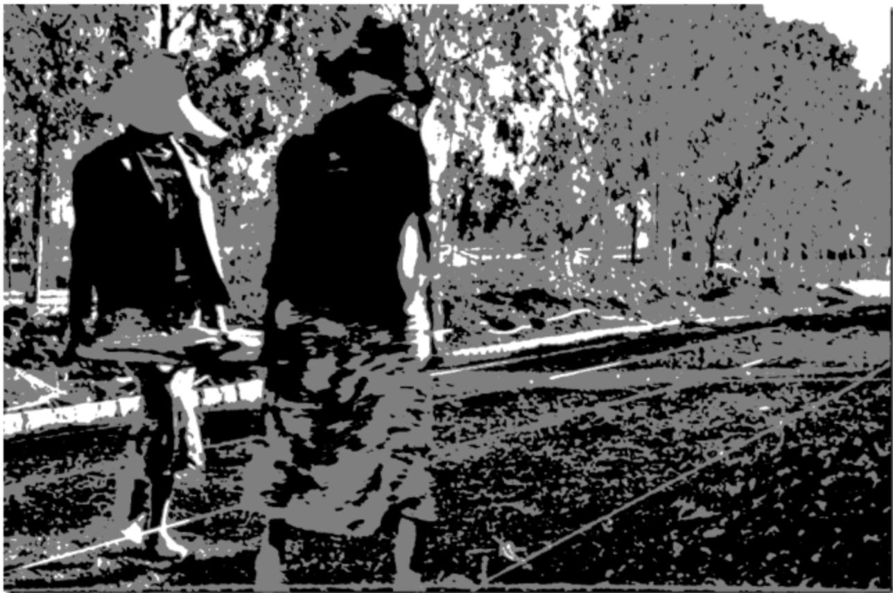
While all steps are critical, the most critical step is securing the edges of the road properly. In this step the worker is digging the supporting trench that will serve as the wall of the road:
